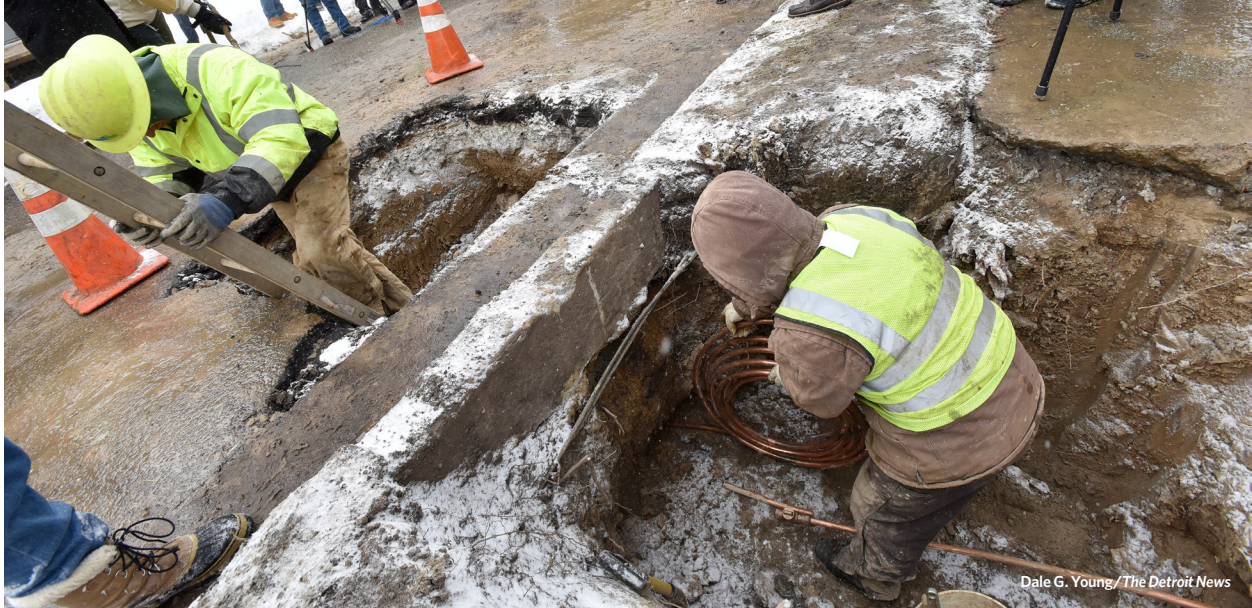
Lansing Board of Water and Light employees replace the last lead service line with copper pipes in Lansing, Michigan, on Dec. 14, 2016.
