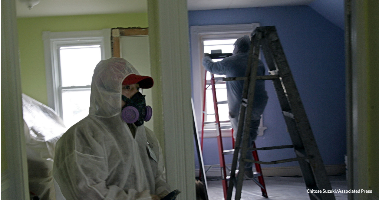
Luis Benitez (left) and Jose Diaz remove lead paint in a contaminated building in Providence, Rhode Island, in 2006.
